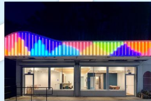
RED'S BEER GARDEN FAÇADE COMPLETED IN 2020
