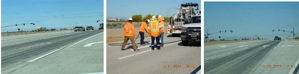
3. Midway Traveled Way Crew – Crack sealing SR98, Group Project crack sealing
