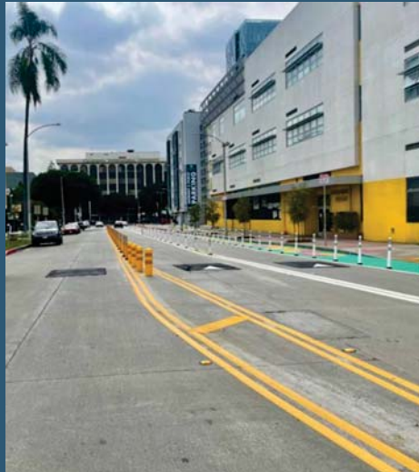
Los Angeles Quick-Build hardened center line, student valet
