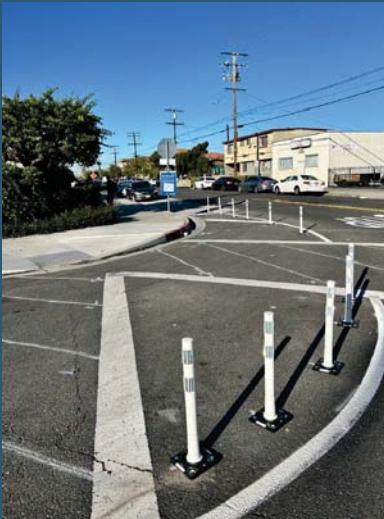
El Monte Quick-Build curb extension
