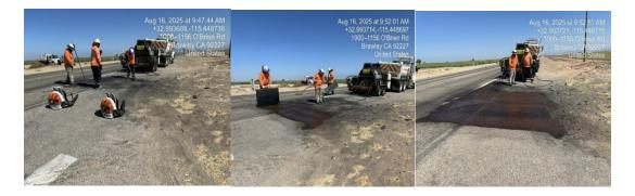
**Pavement Preservation.** Imperial County along I-8 from Imperial County Line (R0.0R) to 98/8 Flyover (R10.3) and 98/8 Interchange. The purpose of this project is to extend the service life of the existing asphalt concrete (AC) pavement by placing a Microsurfacing seal coat. For locations that have damaged AC, the AC will be removed and replaced by a Cold Planing (grinding) operation and the placement new the AC Pavement. Other work includes re-striping, upgrading
