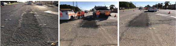
2. The Midway Travelway Crew performed a crack sealing operation on SR-115 to prepare pavement for a scheduled microseal project.
