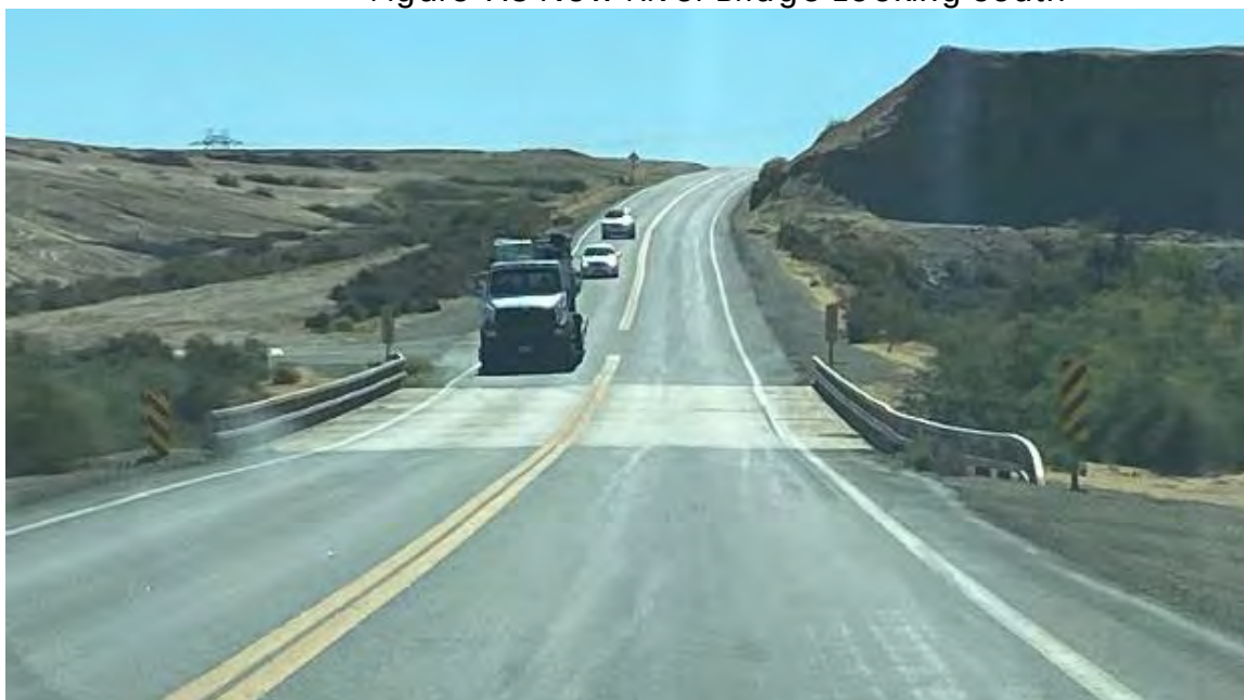
Figure 7.8 New River Bridge Looking South
