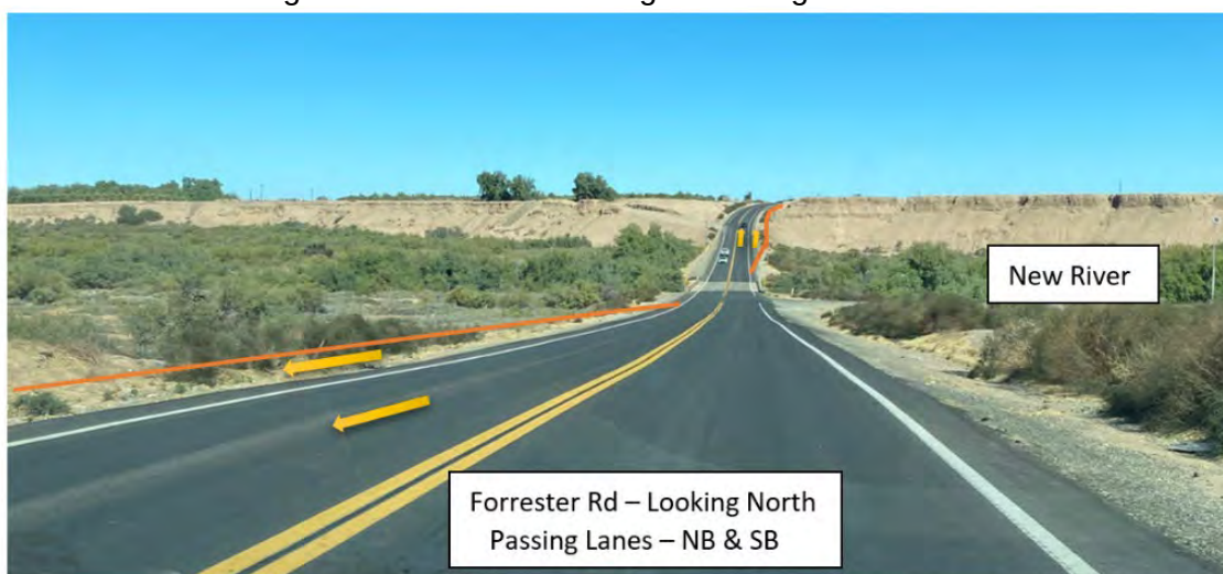
Figure 7.7 New River Bridge Looking North
