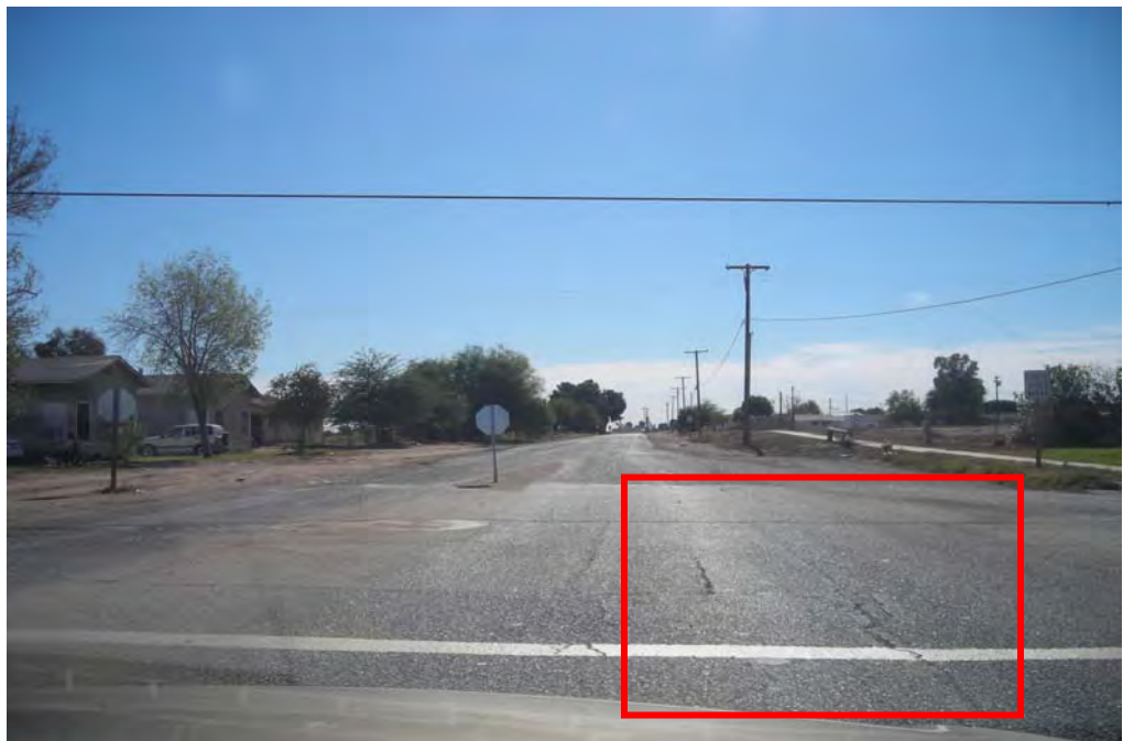
The image above taken at 1 st Street/ Forrester Road illustrates the “rutting” of the roadway.
