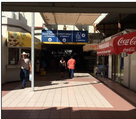
Mexicali I pedestrian tunnel
