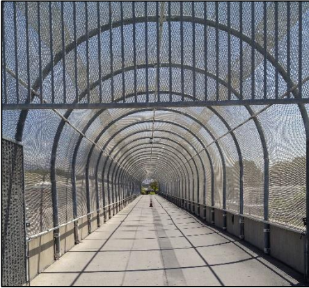
Fencing over existing pedestrian bridge at the Otay Mesa POE
