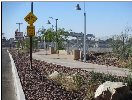
Recently completed pathway project in Andrade
