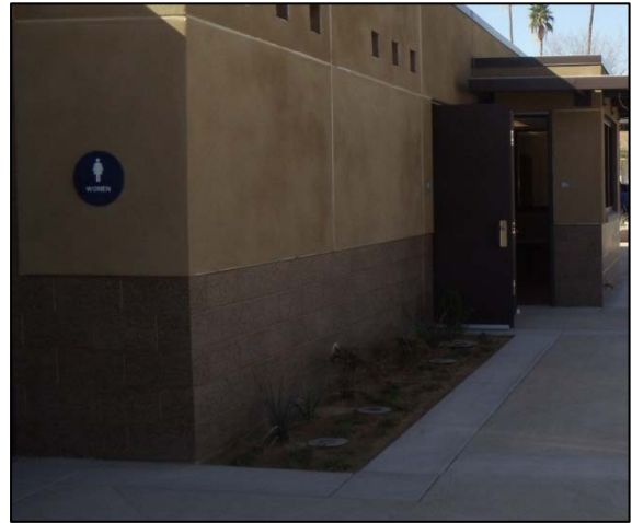
Transfer station restrooms
