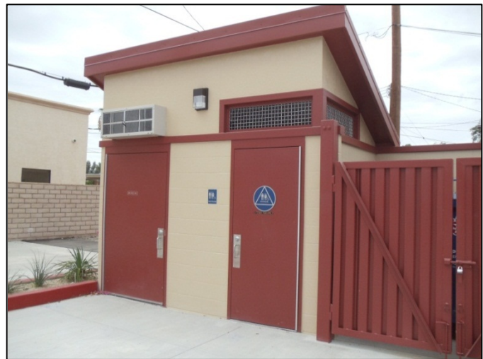
Communications room located in restroom building
