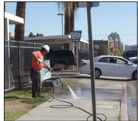
Power washing bus platform
