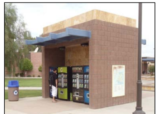
Typical transfer station vending area
