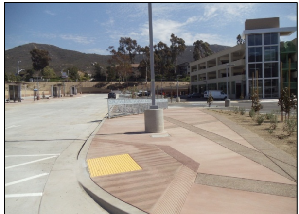
Sabre Springs/Penasquitos Transit Station, where parking is separated from the bus bays
