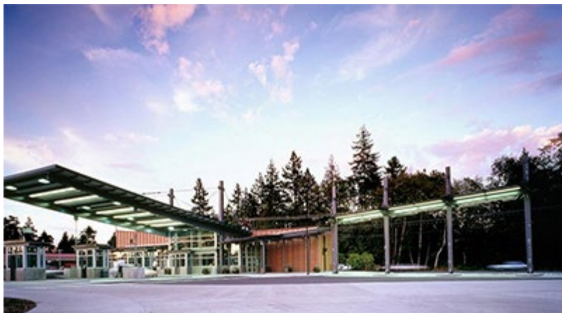
Point Roberts Port of Entry
